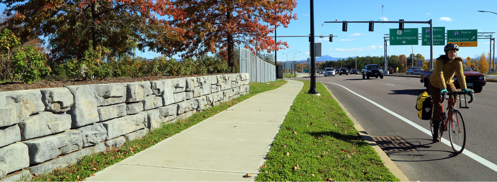
Widening Route 2 at I-89 Exit 14, South Burlington, Vermont
