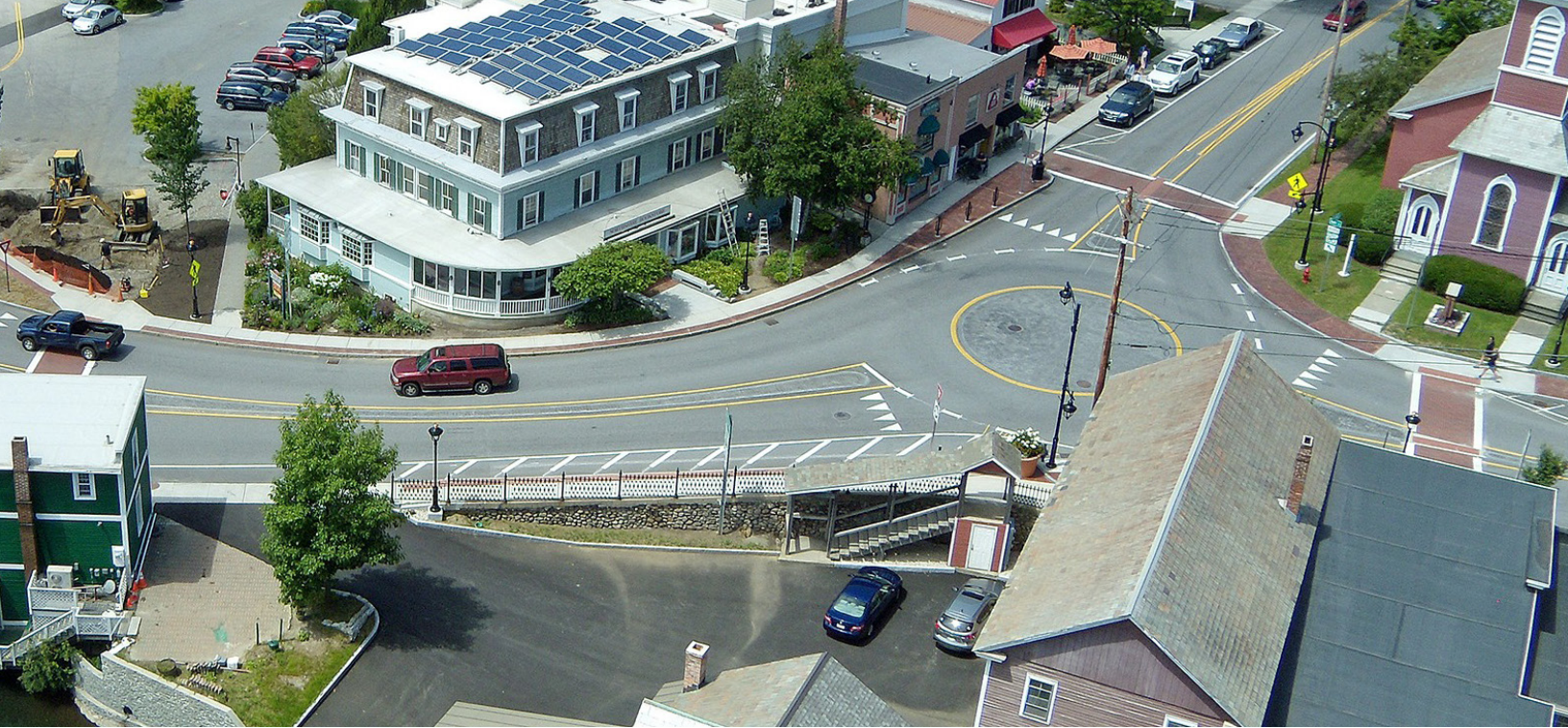
VT Route 7A/11/30 Intersection Improvements, Manchester, Vermont
